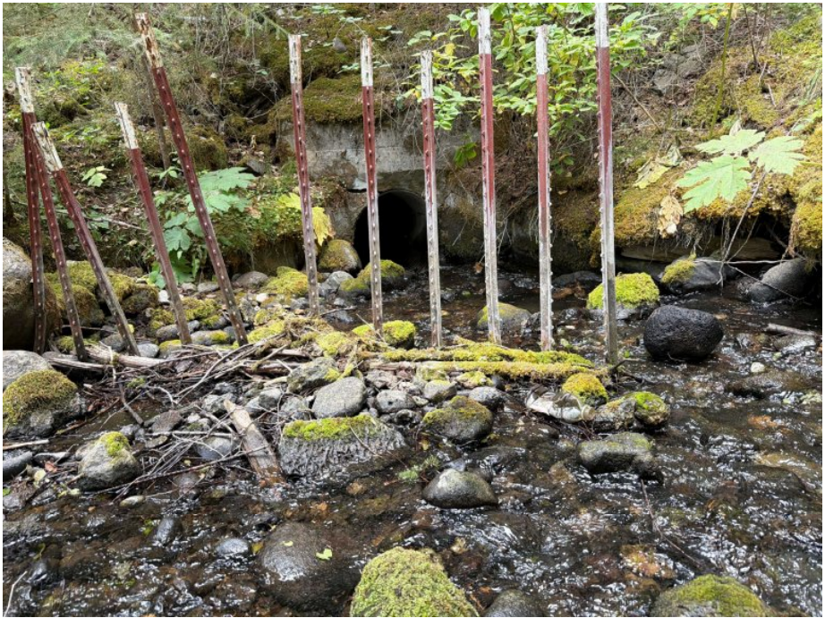
Photo 5 – View looking downstream at the 700mm culvert inlet under the CN Rail embankment. A crude trash rack of angle iron posts has been installed upstream of the inlet; it is unknown who installed the posts.
