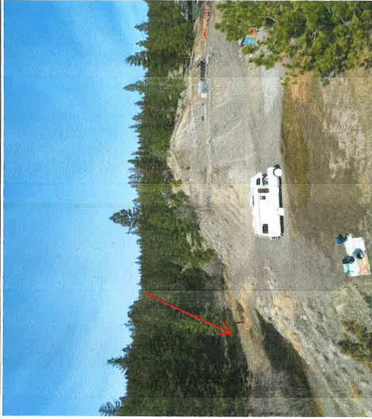
Photo 2: The ravelling cut slopes behind the house on Lot 1 exposing well-drained cobbly sand with trace to some silt, as well as eo
