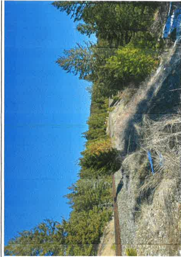
Photo 2: The ravelling cut slopes behind the house on Lot 1 exposing well-drained cobbly sand with trace to some silt, as well as eo
