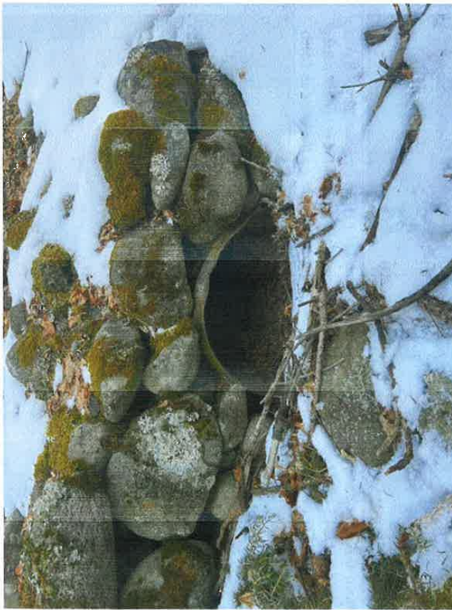
Photo 7: A 400 mm diameter CMP culvert located at the base of the embankment. Debris has infilled approximately 1/3 of the culvert.
