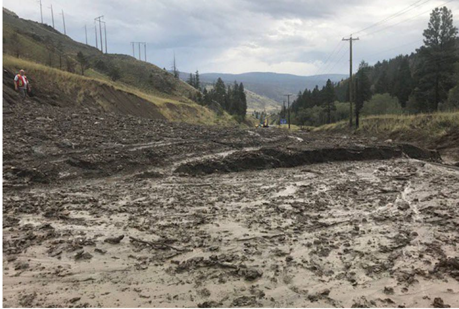
FIGURE 2-1: 2018 MUDSLIDE ON HWY 97 BETWEEN CLINTON AND CACHE CREEK
