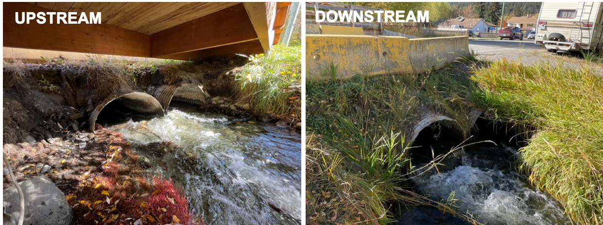
FIGURE 2 CARIBOO AVENUE CULVERTS: UPSTREAM (LEFT), AND DOWNSTREAM (RIGHT)
