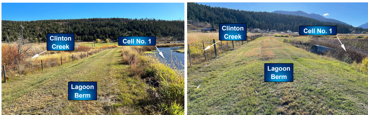
FIGURE 3 WWTP FACULTATIVE CELLS BERMS
