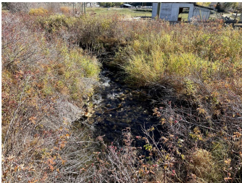
FIGURE 2-3: CLINTON CREEK AT OUTLET OF MACDONALD AVE
