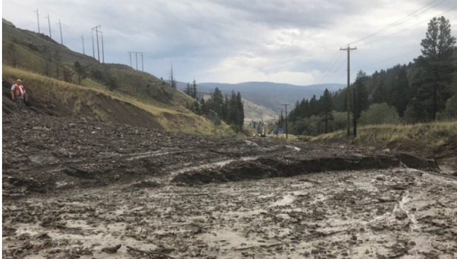
FIGURE 1-4 DEBRIS FLOW BLOCKING HWY 97 SOUTH OF CLINTON, BC (MOTI, 2018/07/31)
