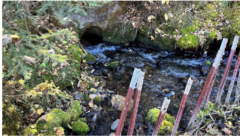
FIGURE 4-3 CN RAILWAY CULVERT
