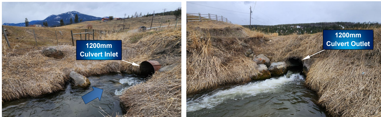
FIGURE 2 CLINTON CREEK CULVERTS AT LAGOON ROAD
