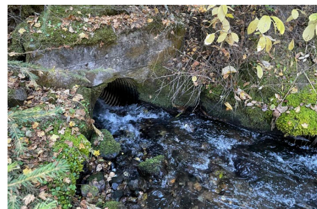
FIGURE 4 700MM CSP CULVERT
