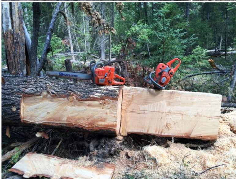
Images: Example of on-site construction of a 34' x 4' bridge with chainsaw ripped 2" decking, by First Journey Trails crew
