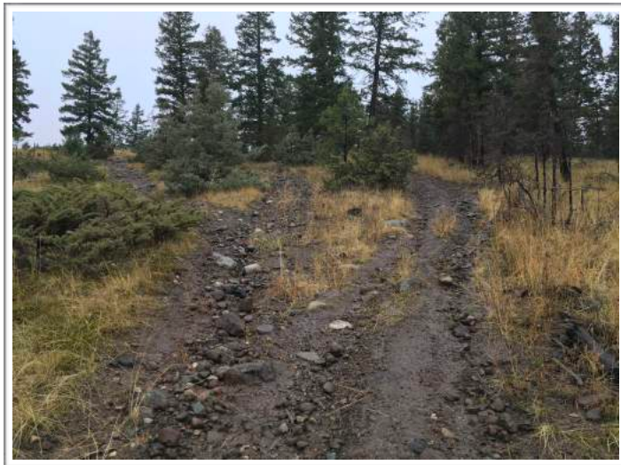
Image: Example of unsustainable trail construction in the Clinton area.
